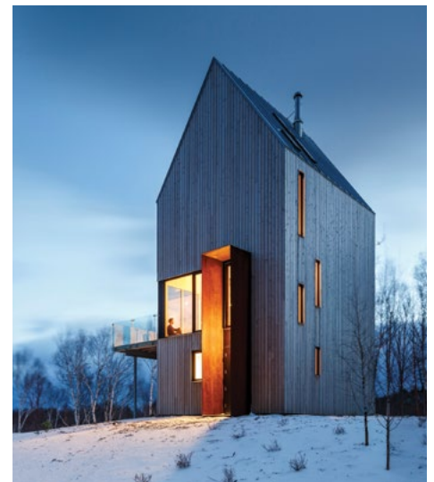
RABBIT SNARE GORGE Omar Gandhi Architect Inc. in collaboration with Design Base 8 (NYC) Photo: Doublespace Photography
